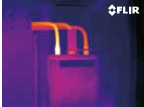
Poor connection and internal damage
