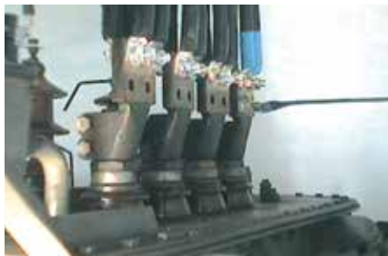
Top of transformer; high-voltage connection.
