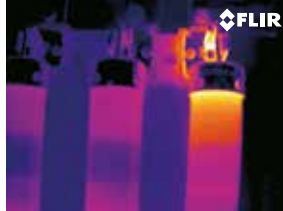
Internal fuse damage
